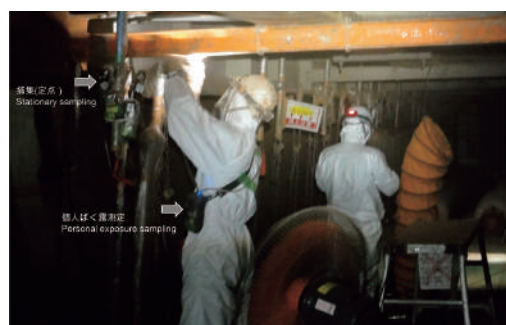
化学物質ばく露による労働災害の原因調査 (道路橋延命工事の鉛入り防錆塗料剥離作業における鉛濃度測定) Exposure monitoring for investigation of an occupational accident (evaluation of lead exposure during removal of lead-containing paint from a steel beam of a road bridge).
