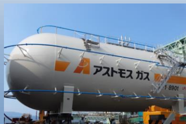
陸上圧力容器 Land Based Liquefied Gas Storage Tank
