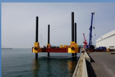
洋上作業台 Self-Elevating-Platform
